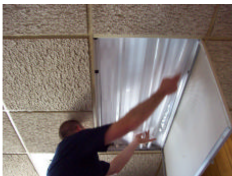
8. Install 2 new T8 lamps
