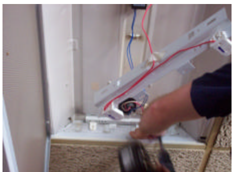
4. Install new T8 socket brackets
