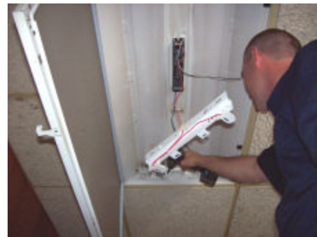
3. Install new electronic ballast
