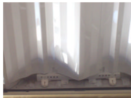
6. Reflector clips on socket bracket
