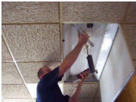
2. Remove ballast & sockets
