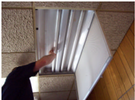
1. Open fixture & remove lamps
