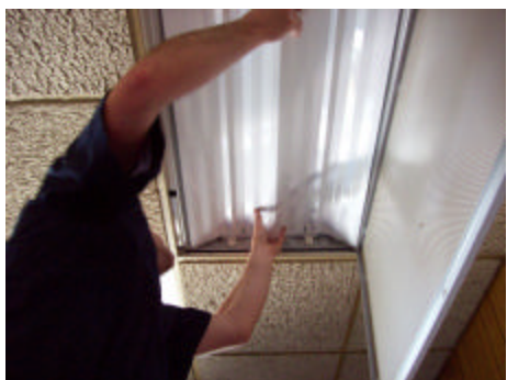
7. Install Best Lights Reflector
