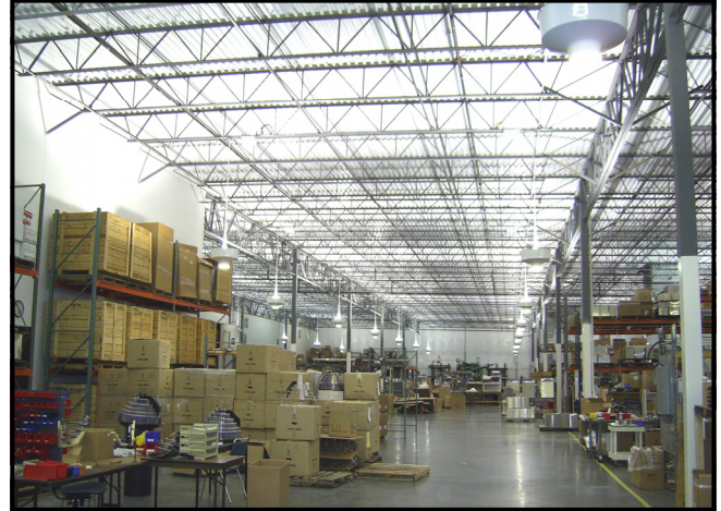
Plant: 62,000 sq. ft. 27' high / 63 -1000 Watt MH-DIA (90% Indirect 10% Direct) spaced 30'x 33' 1.08 Watts per sq. ft. 40 FC
