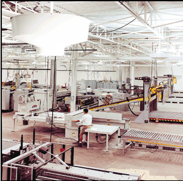
Michigan Box Company; 26,000 sq. ft. with 25' ceiling; 400Watt MH-DIC; 45 FC
