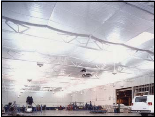
MGA Research*; 20,000 sq. ft. with 27' ceiling; 21-1000Watt MH-IBU; 70 FC 1.05 watt per sq. ft.
